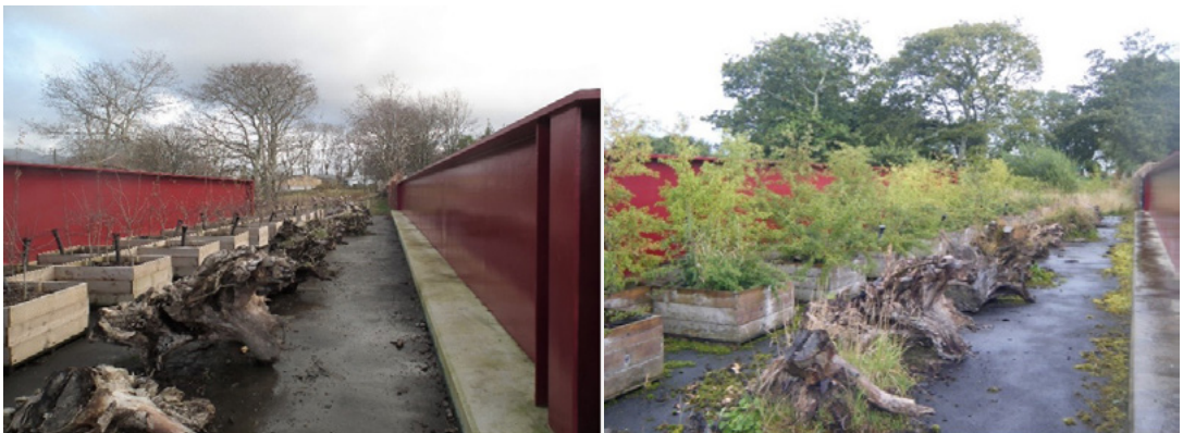
Figure A2.3. Detail of Environmental Overbridge showing shrub saplings in planters and dead wood stumps in 2012 (a) and 2015 (b). © J. Matthews (a, ) © Hyder Consulting (b)
