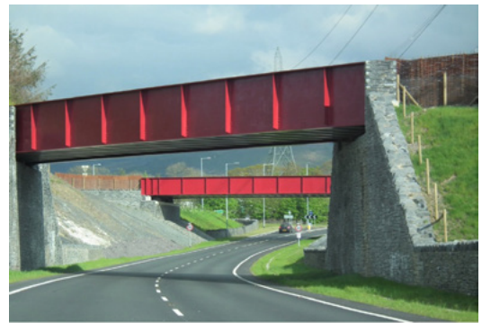
Figure A2.2. Wildlife overpass (foreground) and combined rail bridge and overpass (background). © J. Matthews
