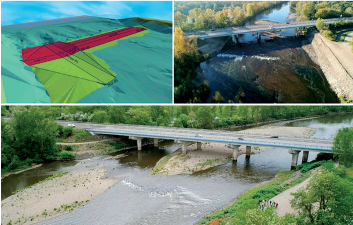
Figure 13 : 3D model of the asymmetric fish ramp. Photographs of Weir A89 after adjustment in 2 distinct periods. ©Vinci Autoroutes
