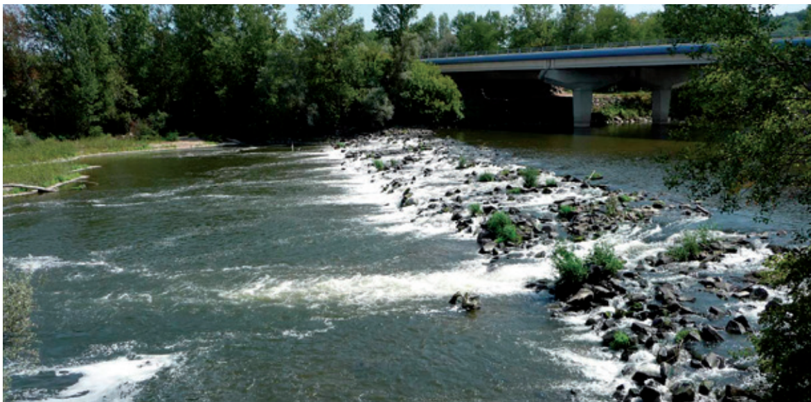
Figure 12 : Photograph of Weir A89 (ROE 63404) before works. ©Vinci Autoroutes
