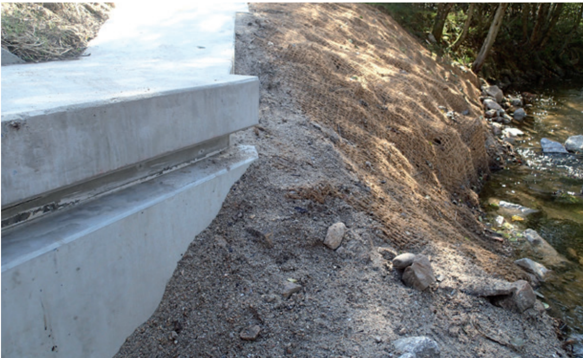
Photoset 1: Illustrations of the structure and its remodelling for small wildlife (photos taken during the construction phase). © GREGE Up: View of the Deiro structure - Down: View of the wildlife footway and hollered out "micromammals" section created and access to the downstream riverbank.
