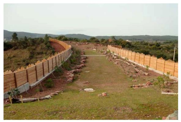
Figure 2.2. Wildlife overpass with several measures providing shelters that favour its use by small animals. Photo: S. Vanpee - IRSTEA.
