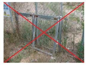
Figure 15.11. Swinging escape hatches for medium-sized carnivores, permanently open because its hinges have rusted, allowing animals to enter the fenced area. Photos: F. Navàs.
