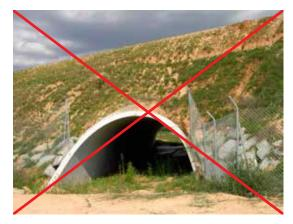
Figure 6.10. Incorrect fencing of the underpass walls permits animal access to the embankment. Photo: C. Rosell.
