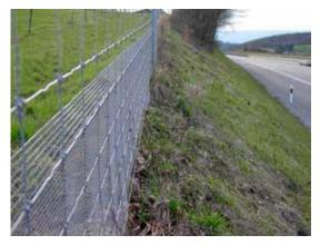
Figure 14.2. Reinforcement on the non-road side of conventional mesh. Photo: C. Rosell.
