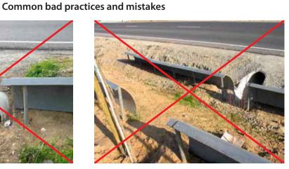
Figure 11.11. Discontinuity between different sections of the guide fences. Photo: F. Navàs.
