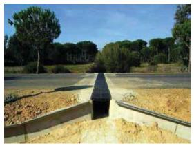
Figure 11.3. Amphibian crossing with funnel-shaped guide structure. Photo: GIASA.
