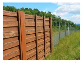
Figure 2.5. Screens on crossings must be in perfect continuity with the road perimeter fence. Photo: C. Rosell.
