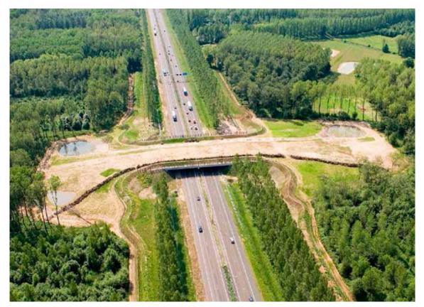
Figure 12.2. Adaptation of ecoduct entrances, combining patches of soil and rows of branches that provide shelter and lead the animals towards the structure. Ponds also attract wildlife. Photo: H. Bekker.
