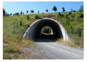
Figure 7.4. Unpaved track and fence tied in with the underpass wing walls encourages wildlife usage. Photo: M. Fernández Bou.
