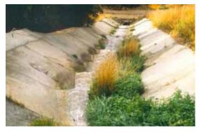
Figure 9.8. Protective culvert outlet on an embankment with sloping side walls adapted to facilitate movement by wildlife. Photo: C. Rosell.
