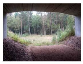
Figure 6.3. Natural soil underpass base. The lack of light and moisture do not allow vegetation growth inside the structure. Photo: C. Rosell.
