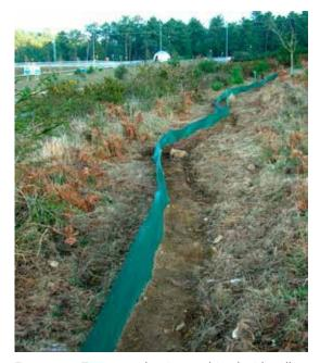
Figure 11.8. Temporary barrier combined with collection buckets. Photo: Environment Office, University of Vigo.
