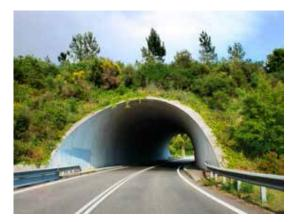
Figure 2.3. Wildlife overpass located in a section between cuttings, enabling excavated earth to be recycled. Photo: M. Fernández-Bou.
