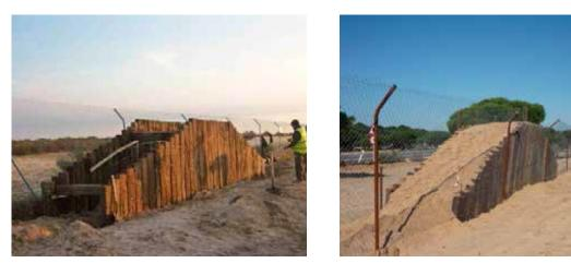
Figure 15.5. Escape ramp. On the left, viewed from the road side during the construction process, and right, viewed from the outside, once completed. Note that the fencing mesh has been removed at the top of the ramp to make it easier for animals to jump across. Photo: Public Works Agency. Government of Andalusia.
