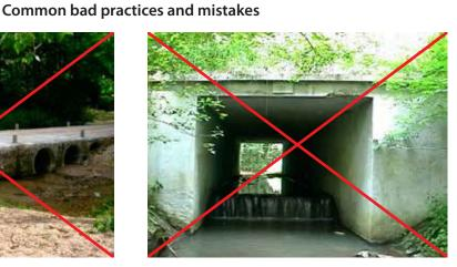
Figure 10.3.Step inside a culvert hindering the movement of aquatic fauna. Photo: J. Dufek.
