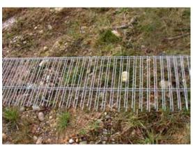
Figure 13.6. Detail of welded wire mesh reinforcement. Photo: C. Rosell.
