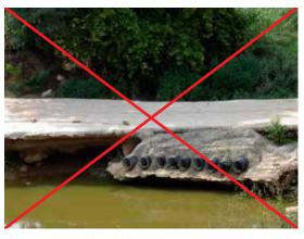
Figure 5.6. Works track that has interrupted the continuity of the watercourse. Photo: R. Campeny.
