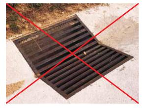
Figure 20.5. Manhole and drain gratings must be dense to prevent small animals from falling inside. The walls of these structures should also be adapted to help animals to escape. Photo: C. Rosell.
