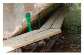
Figure 9.5. Platform that facilitates animal movement through a culvert. Photo: Development and Environment Department, Government of Castilla y León.
