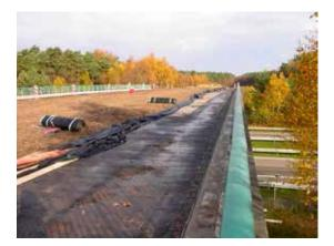
Figure 2.7. Wildlife overpass insulation and surface drainage. Photo: C. Rosell.
