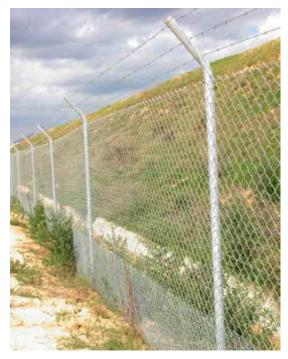
Figure 14.3. Fence combined with an outrigger to prevent deer from jumping over and base reinforcement for small vertebrates. Photo: M. Fernández Bou.
