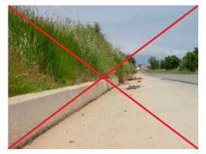
Figure 20.4. Vertical kerb wall: a barrier for small animals that fall onto the road and cannot escape. Photo: C. Rosell.
