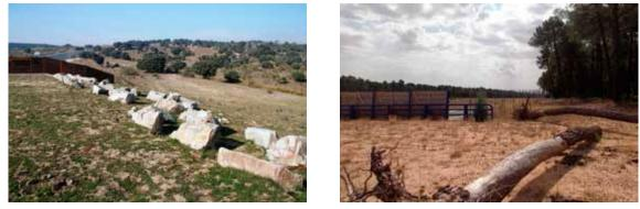
Figure 1.11. Two alternative systems using boulders and tree trunks to avoid vehicle movement across the ecoduct. Another option is to install metal or timber barriers at a suitable height and signs prohibiting vehicular traffic. Photos: Javier Cantero and CEDEX.
