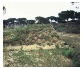
Figure 15.3. Escape system consisting of an vegetated soil ramp, seen from road side. Photo: H. Bekker.
