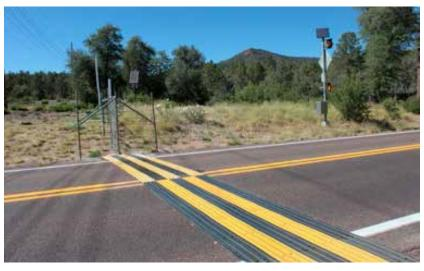
Figure 15.9. Electrified mat preventing animal entrance to a fenced main road via a paved access track. Photo: C. Rosell.
