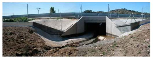
Figure 11.7. Fence leading amphibians towards a wildlife crossing under construction. Photo: Javier Cantero.
