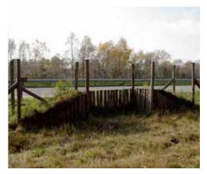
Figure 15.1. Ramps designed to allow roe deer to escape from inside a fenced section. Photo: C. Rosell.
