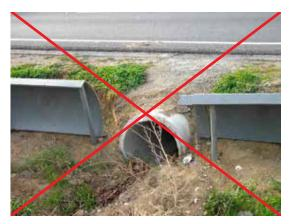
Figure 11.10. Maladjustment between guide structure and amphibian crossing entrance. Photo: C. Rosell.
