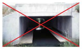
Figure 9.10. Lack of ramps connecting the dry ledges with the adjacent areas. Photo: F. Navàs.
