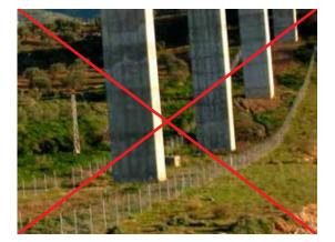
Figure 5.9. Long section of perimeter fencing under a viaduct which prevents animal passage. Photo: Minuartia.
