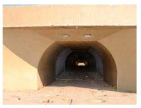
Figure 11.2. Interior of an amphibian crossing with a semi-circular section. The vertical walls and the flat base facilitate amphibian movement. Photo: M. Puky.
