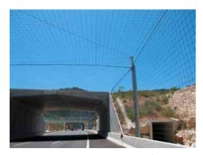
Figure 14.5. Polyamide net structure in a funnel shape to prevent bat collisions on a highway, with hitherto inconclusive results. Photo: M. Fernández Bou.
