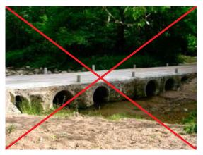
Figure 10.2. Drains located on a ford, hindering fish movements. Photo: F. Navàs.
