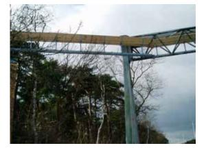
Figure 4.2. Timber platforms installed on a motorway sign post. Photo: H. Bekker.
