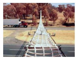
Figure 4.3. Mesh bridge crossing. In areas with a high fire risk, fire-resistant material must be used to prevent propagation. Photo: Kylie Soanes.
