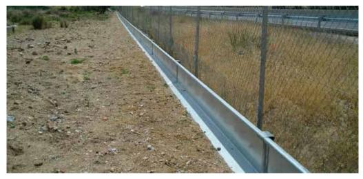
Figure 11.6. Opaque metal structure applied to a fence to guide amphibians towards the crossings. Photo: CEDEX.
