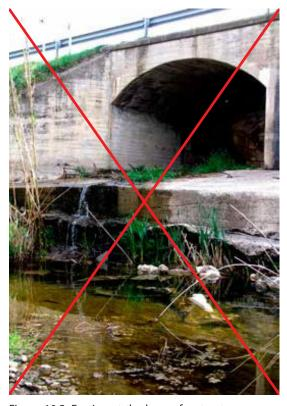
Figure 10.5. Erosion at the base of a structure, generating an insurmountable obstacle for aquatic fauna. Photo: M. Clavero.
