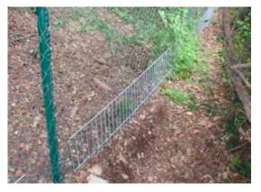
Figure 13.5. Wild boar reinforcement in a particularly troublesome section. Photo: Túnels Barcelona-Cadi.
