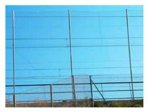
Figure 14.4. Fencing 5 m high and simple chain-link to avoid bat collisions on a high-speed railway line. Photo: ADIF.
