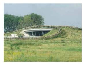
Figure 2.4. Wildlife overpass located on flat land, with access ramps on a gentle slope. Photo: P. Farkas.
