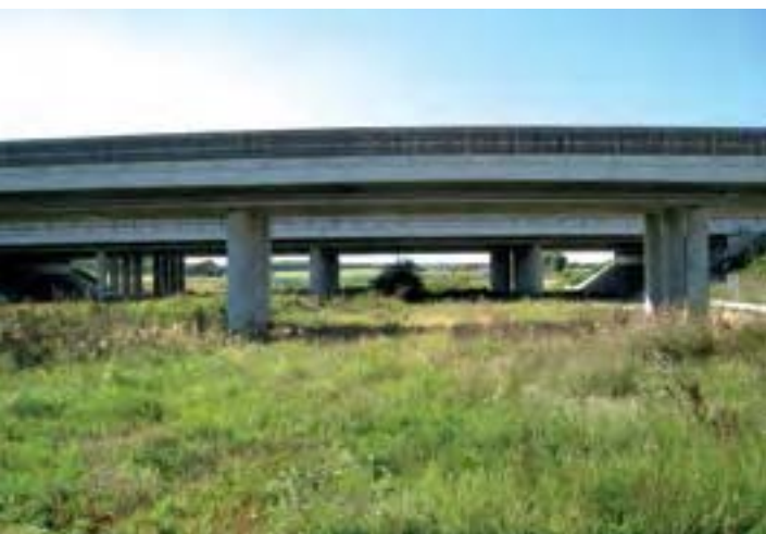
Measures in favour of ecological connectivity along a highway in the Alps-Carpathians-Corridor area visited by the members of the Platform Ecological Network.
