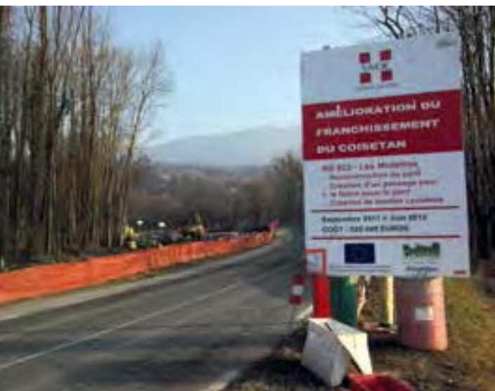
The corridor contract for the area of the ecological corridor linking the Nature Park Massiv des Bauges and the Nature Park Chartreuse foresees various measures pertaining to existing water courses, like here the building of an under-path at a bridge crossing the Coisetan river.
