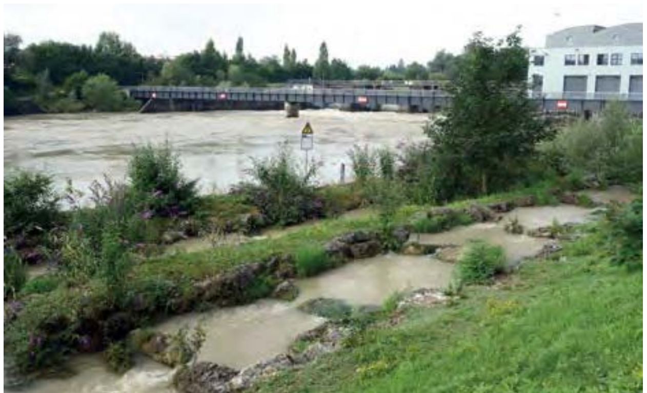
Example of a specific connectivity measure: fish ladder near Olten in the Canton of Solothurn (Switzerland).
